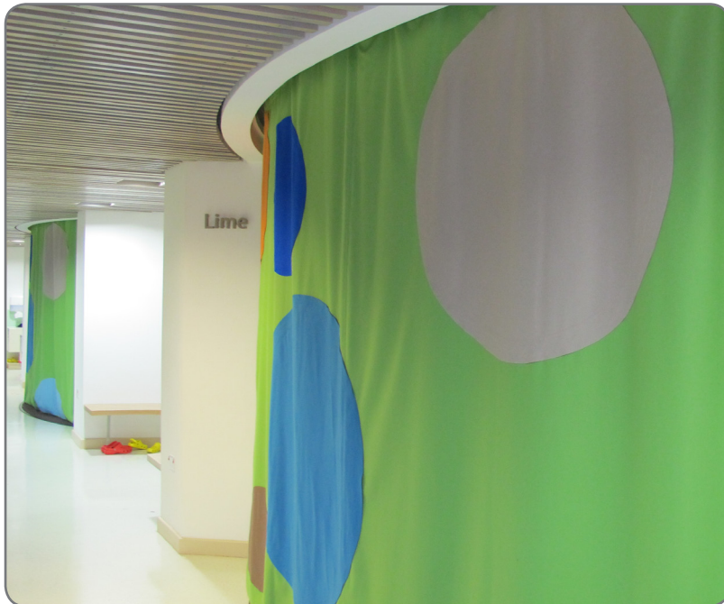
Bespoke acoustic drapes act as the dividing walls between the classrooms in Hartlepool's Jesmond Road Primary School.
