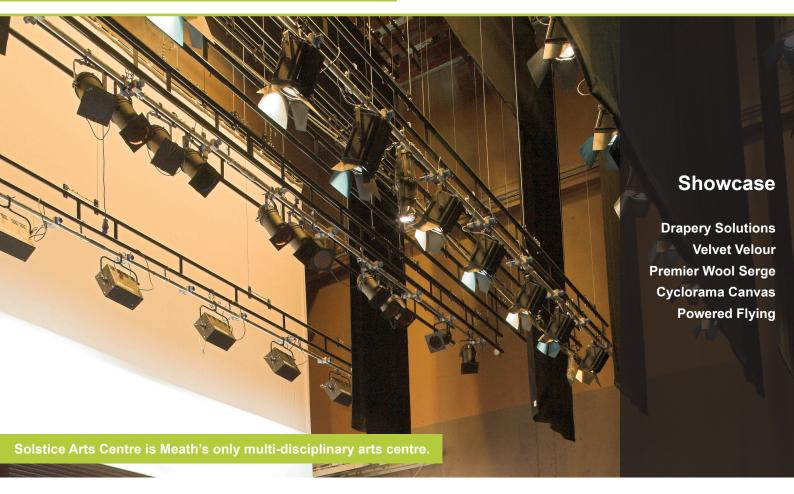
J&C Joel installed pilewind winch units, rigging equipment and stage dressings within the main auditorium of the Solstice Arts Centre in Navan, County Meath, the Republic of Ireland.
