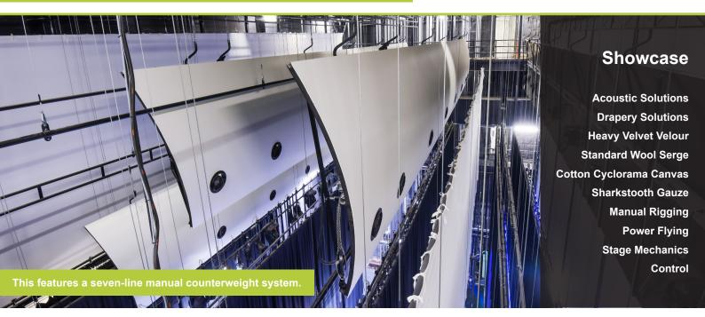
In one of the company's largest installations to date J&C Joel carried out a complete fit out of Zayed University's Abu Dhabi campus auditorium installing a complete rigging system, stage dressings, stage machinery and an acoustic shell for the venue's stage.
